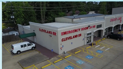
Emergency Hospital Systems- The Woodlands 20225 Interstate 45 N. Spring, Tx 77386
